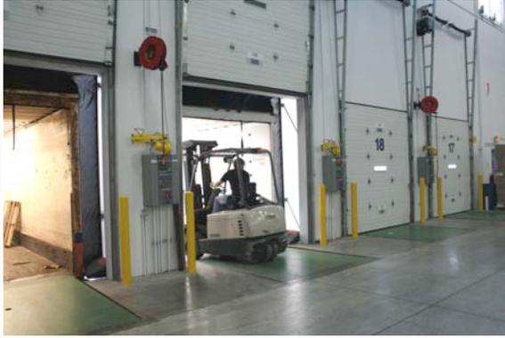
They sequenced all of these components so there is a domino affect - the restraint secures the trailer, then the door opens, which then allows the leveler to operate, and lastly the dock light turns on.
